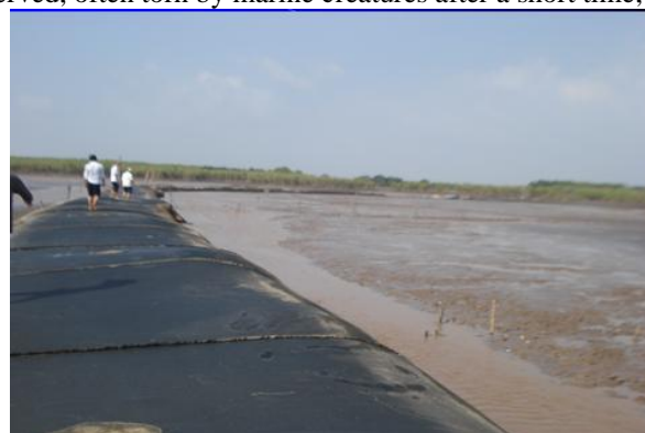
Figure 18. Wave collection by Geotube at Nha Mat in Bac Lieu province has no effect on wave deceleration due to the crest has been lower than the 1.2 m design.
