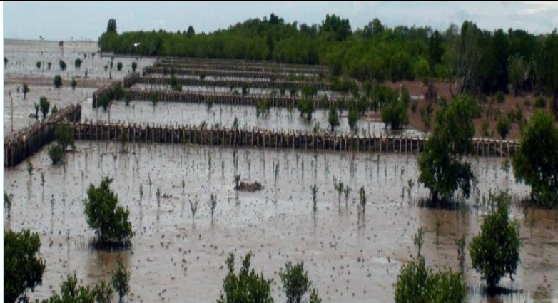
Figure 19. The fence for beach feeding and rehabilitating mangrove forests in the GIZ project in Bac Lieu,
