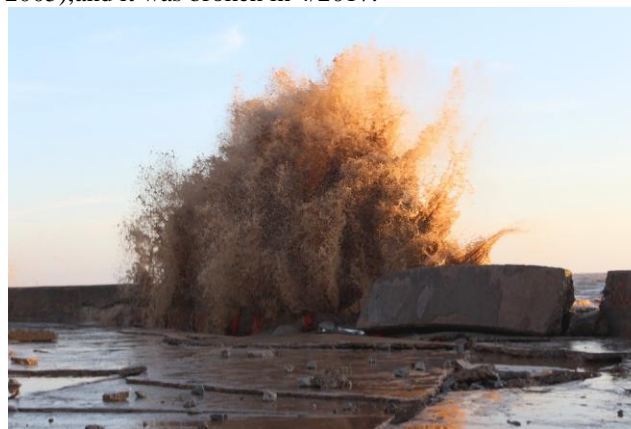
Figure 16. The protection of Ganh Hao town in Bac Lieu province broken by waves in 4/2017 (source: tuoitre.vn)
